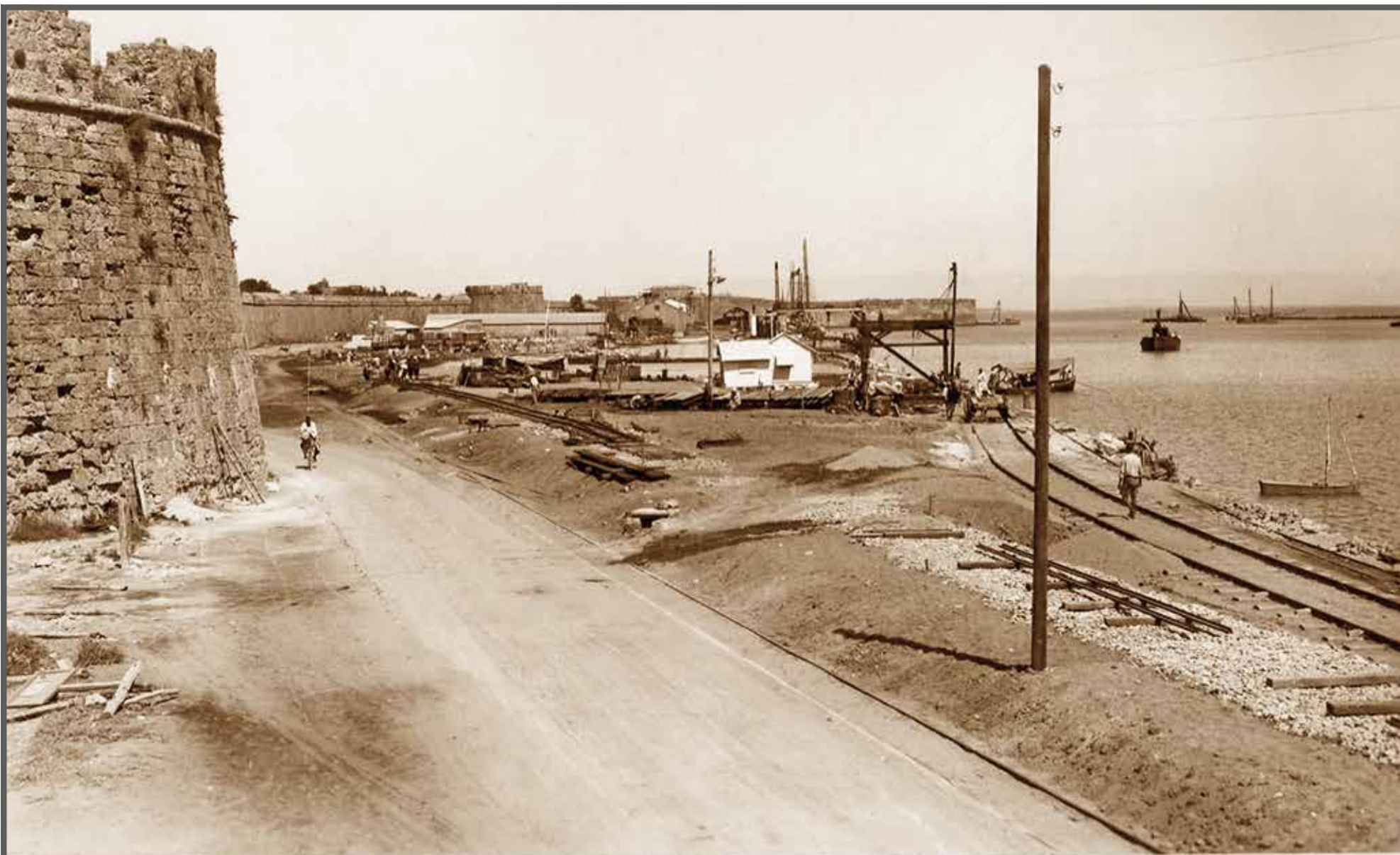
Reclamation, from end of old glacis now removed, showing track laying, and ends of drains to Ditch and Arsenal Gate - 3 rd Aug. 1932.
